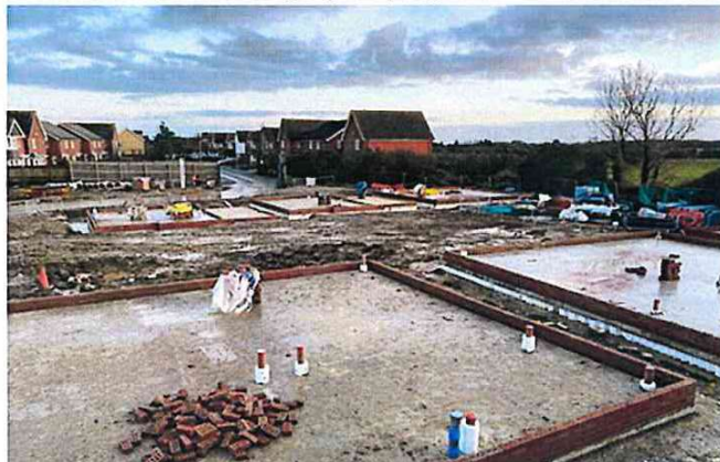
Puffin Road, Hillborough (site progress – foundations laid)
