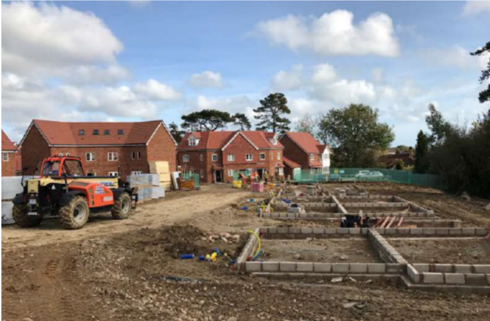
Hailsham: construction work in progress on phases 2 & 3
